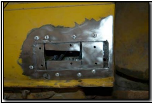
Rivets popped into place
