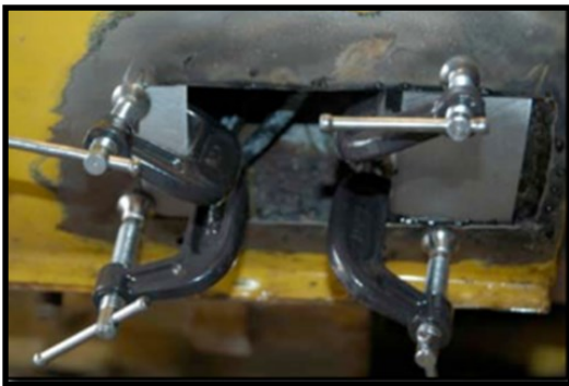
Flanges are clamped into place
