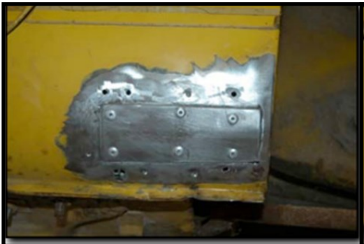
Plate inserted and riveted into place
