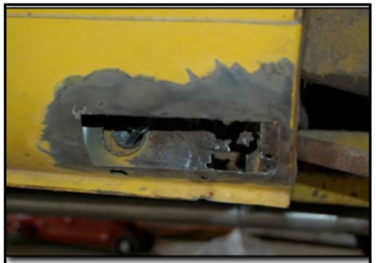
Bad metal is cut out and hole is squared off
