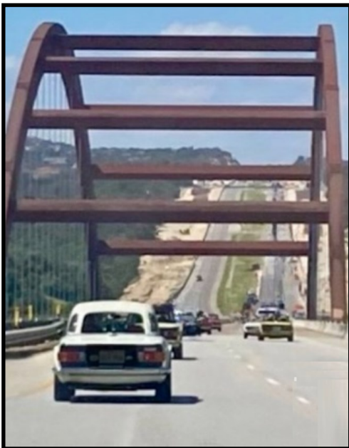
A long line of Triumph's crossing the Lake Austin bridge on the way to the picnic
