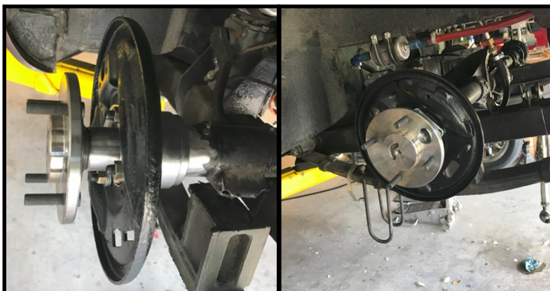
Figure 7 & 8: Test fit and Tack Welded. Note: The hole in axle flange for putting a socket through, you have to request this when ordering.
